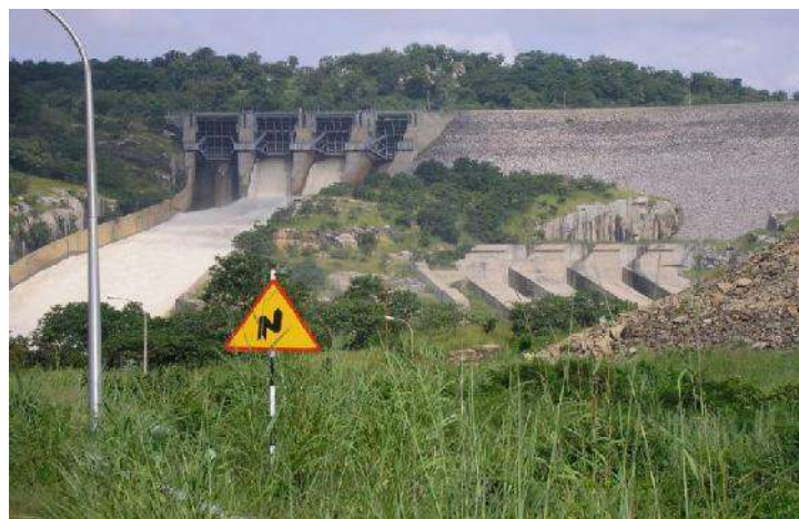
Fig. 1: Spill gates & Penstock of Shiroro Power Station.
