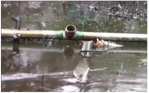
Plate 5: Typical Crude Oil Tapping Point
