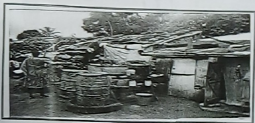
Plate 5: Bad roof condition
