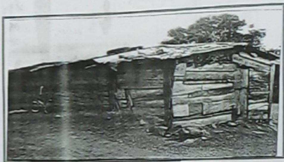
Plate 3: Make shift structure.
