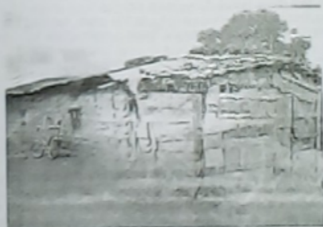
Plate 3: Make shift structure
