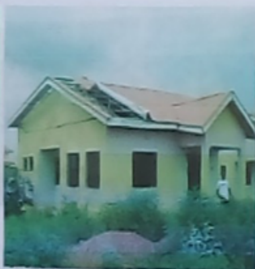
Plate 3: Cracked wall Source: Authors field work, 2010
