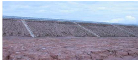
Plate 1; Typical view new railway in Nigeria
