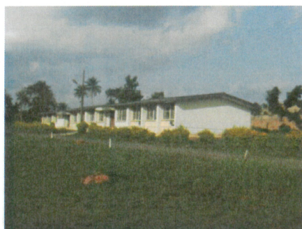
Plate 3: Pictorial View of Rehabilitation Centre for the Disabled, Moniya, Ibadan Source: Researcher's Field work, August, 2018
