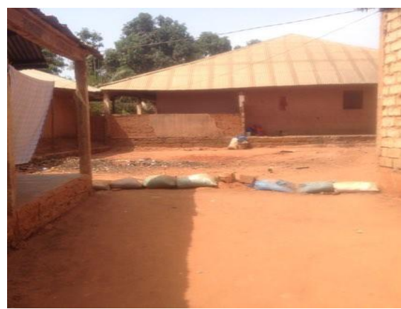
fig.2 roof: corrugated zinc sheets
