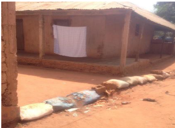
fig.3 earth bags against floods
