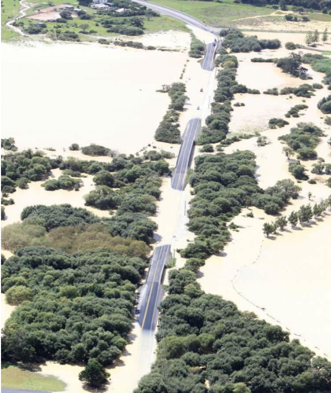
Figure 5: Flooding at Kawakawa Triple Bridges in July 2014 (looking north)
