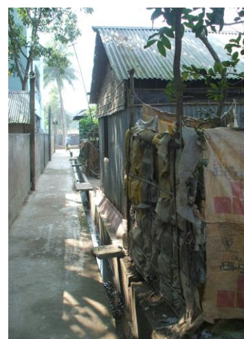
Figure 2: Paved walkways and drains built by LPUPAP in a slum in
