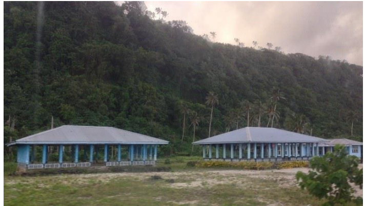
Figure 3: Remaining, abandoned Tsunami houses in Lepa (Image Author's Own)
