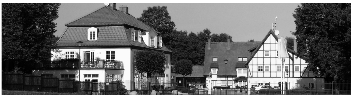
Figure 4: Buildings from complex „ Dwór Oliwski”, in Poland
