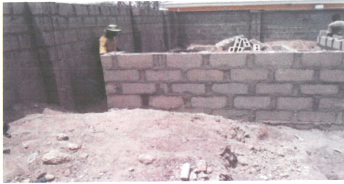
Plate 7: Showing Recent construction works at Bosso Estate Minna with less than 600mm setback from the left-side, right and rear sides of the Fence. (Source Researcher's field work 2011)
