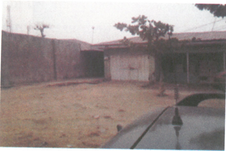
Plate 5: Showing Building along Bosso Road Minna with 1.4 m Side-Setback between Buildings of different compounds whereby eave of one building encroaches into the next compound. (Source Researcher's field work 2011)
