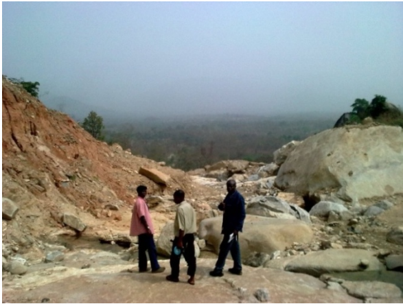
Figure 3. Photograph of major landslide out of the fourteen that occurred in the area
