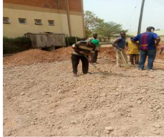
Figure 6: Dry mix of soil, cement and CCR
