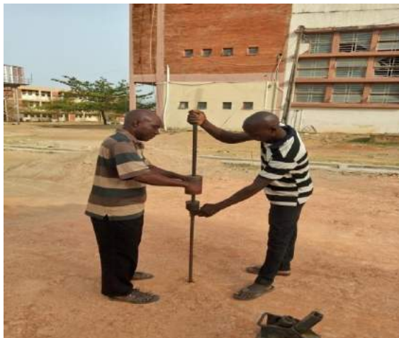
Figure 10: Dynamic Cone Penetration test on Finished Road Surface
