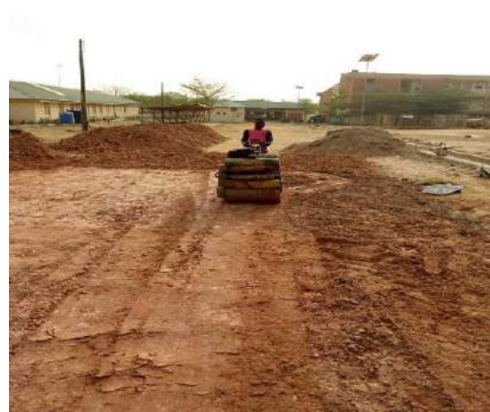
Figure 7: Compaction with light roller
