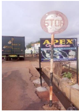
Figure 3 Signage at 0+075m on Murtala Moh'd Rd
