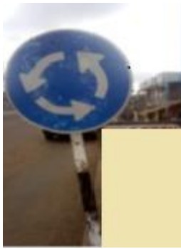
Figure 1 Signage at 0+145m on Unity Rd
