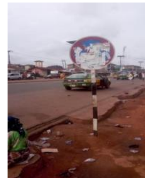
Figure 7 Signage at 1+038m on Murtala Mohammed Rd
