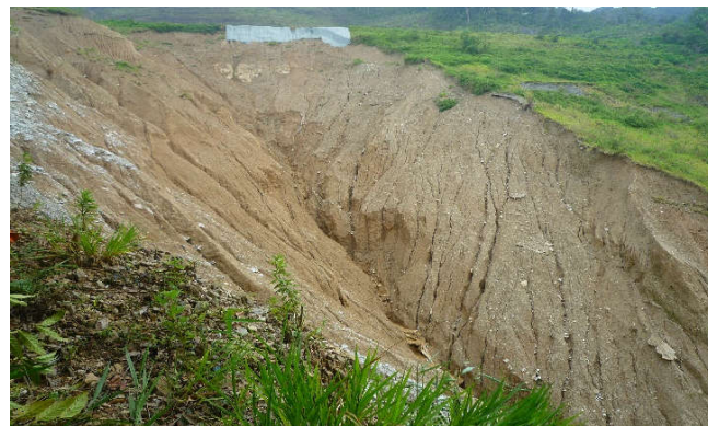
Fig. 1. Landslide event at Cameron Highland, Malaysia.
