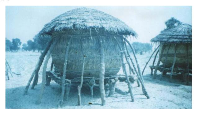
Plate 4: Thatched Rhombus with tree stem columns, showing tree stem external support Source: adapted from (Adejumo & Raji, ibid)
