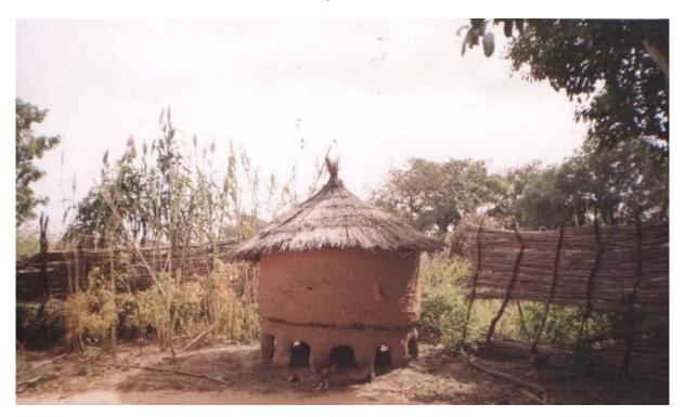
Plate 3: Mud Rhombus with stone grillage foundation floor assembly and thatched roof Source: adapted from (Adejumo & Raji, 2007)
