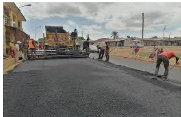
Figure 7 Asphalt Pavement of Emirs' Road Kaiama Round About, Patigi
