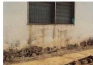
f) Water run marks on window
