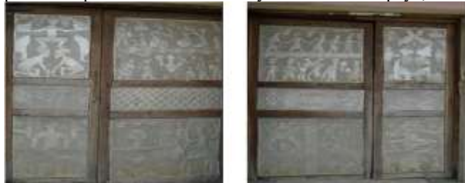
Figure 16: Entrance Doors Fieldwork, 2022
