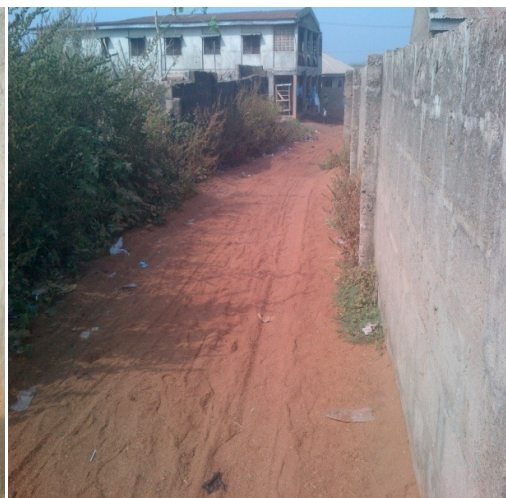
Plate 8: Filled Road Ditches
